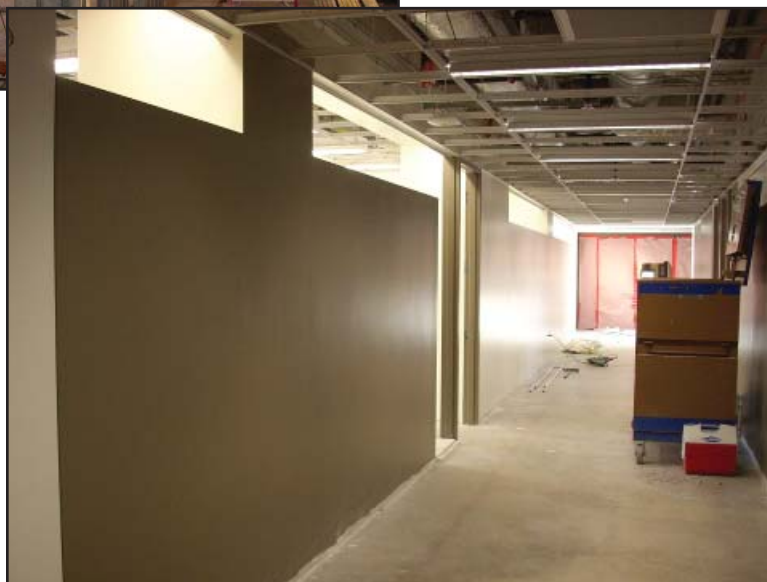
3/25/11 - (right) Painting is complete and barriers have been pulled down.
